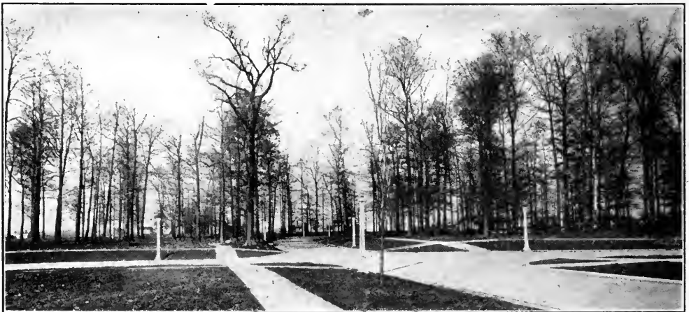
A STREET INTERSECTION AT FOREST PARK, KOKOMO, IND. Note the fine trees and the sidewalk built around one of them
